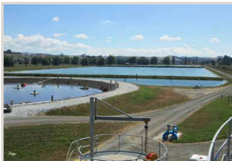
OVERVIEW - TE KUITI WASTE WATER TREATMENT PLANT
