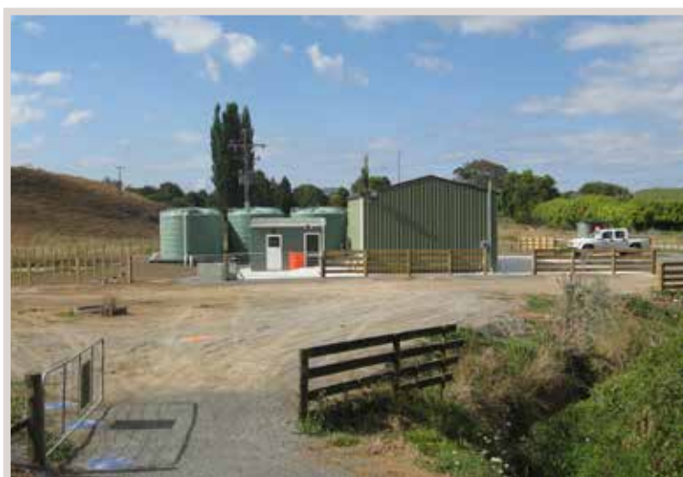
PIOPIO WATER TREATMENT PLANT
